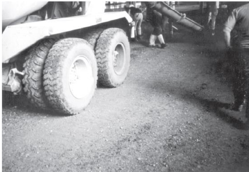
Figura No. 4 “Proof- Rolling Test” (ACI 302, 2015)
