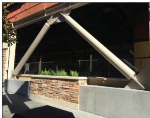
Figura 4. Riostra CoreBrace. No.11, N. S. (2015). Seismic Design of Steel Buckling-Restrained Braced Frames
