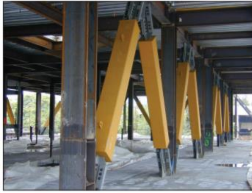
Figura 5. Riostra Nippon Steel, No.11, N. S. (2015). Seismic Design of Steel Buckling-Restrained Braced Frames
