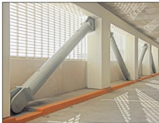
Figura 6. Riostra Star Seismic, No.11, N. S. (2015). Seismic Design of Steel Buckling-Restrained Braced Frames
