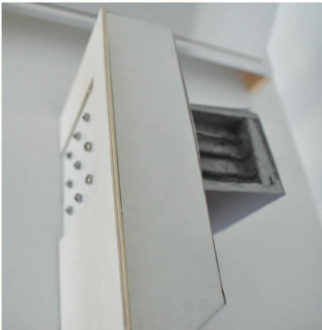
PLACA DE ACERO Y VIGA SOSTIENEN LA FACHADA EXTERIOR
