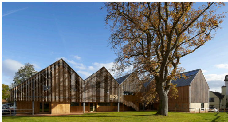
Figura 9. Fachada de la escuela Bedales School Art and Design. (ArchDaily, 2016)
