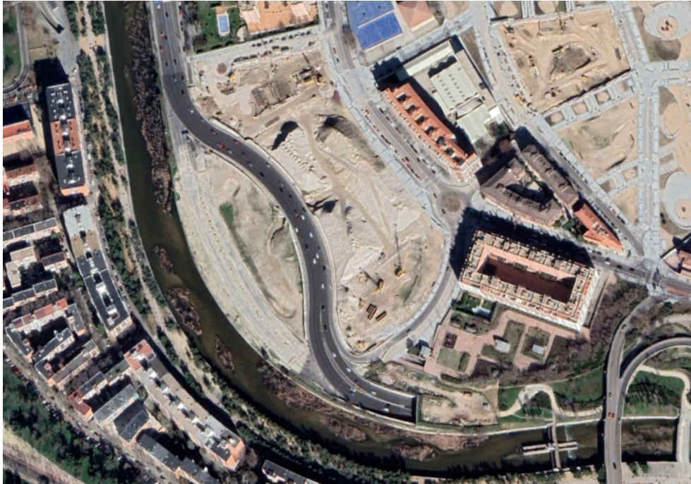
Figura 6. Lote a intervenir. Goggle Earth.
