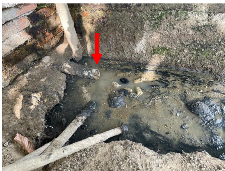
Figure 6. Drainage of pig pens in one of the family units. The water that is coming out of the barn can be seen to be puddled outside and the formation of sludge can be seen.
