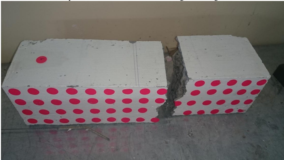
Fig. 15: Failure pattern for beam 6 at the side of the camera
