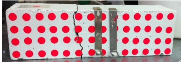
Fig. 7: Failure pattern for beam 3 at the side of the LVDTs.
