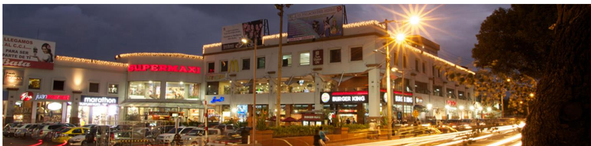
Figura 7. Fachada principal CCI
