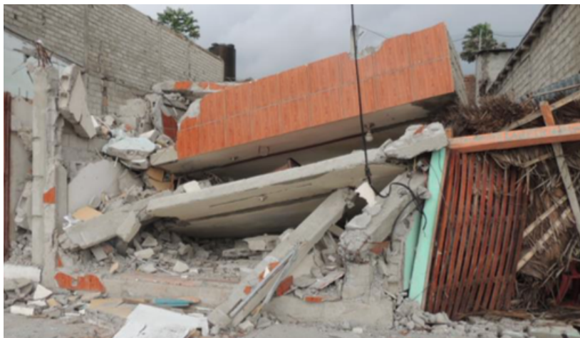
Figura 65. Losa plana (GEER, 2016)
