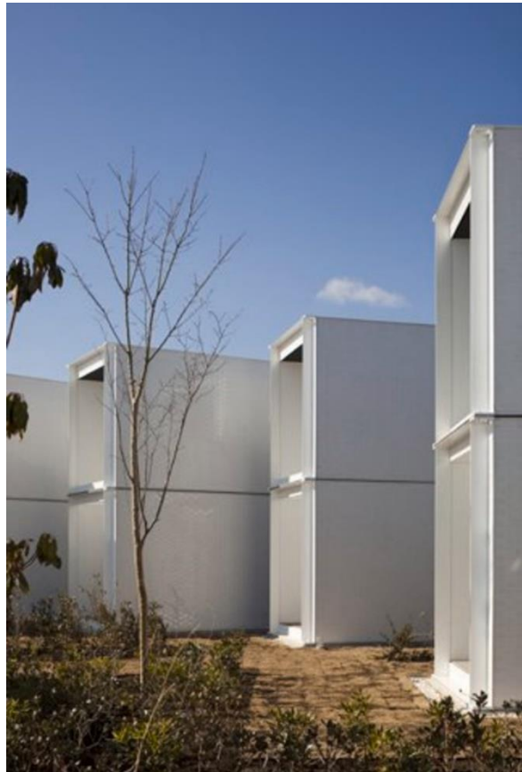
Figure 12 Hotel Bayside Marina
